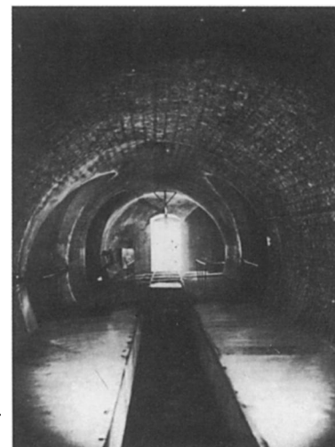
4. Photograph by Félix Nadar of the Paris sewers, 1865.
